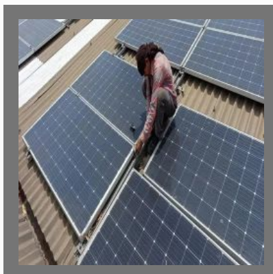
Solar Power Plant Installation Service
