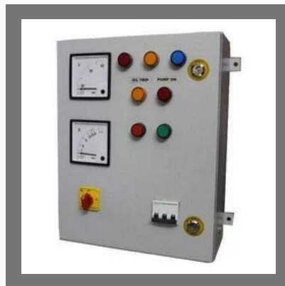
Three-Phase Control Panel
